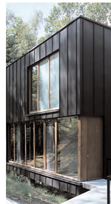
Individual Housing, Villiers-La-Ville (Belgium) Architects: Stekke & Fraas
