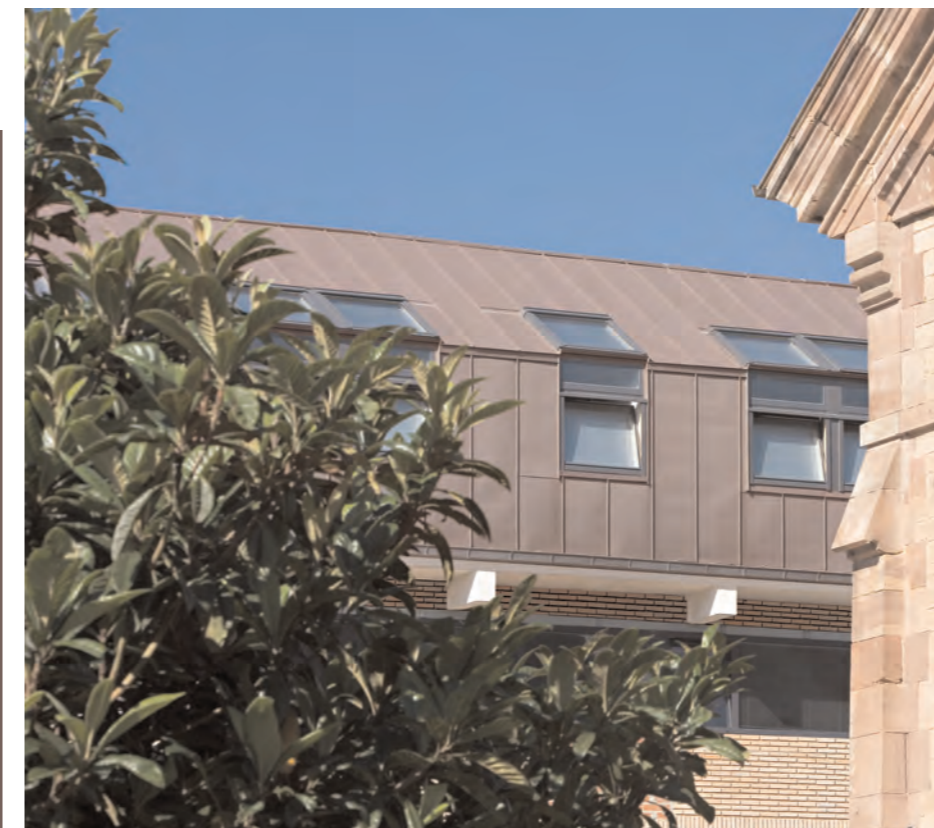
Retirement home, Carrejo (Spain) - Architect: Carlos Navarro
