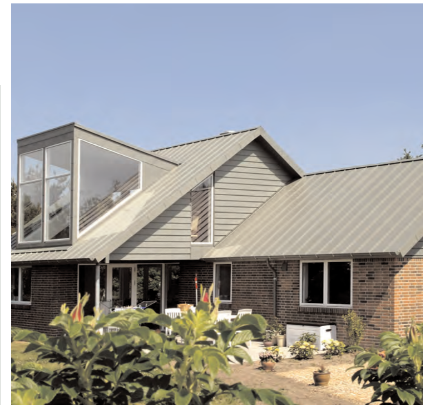
Individual housing, Odder (Denmark)
